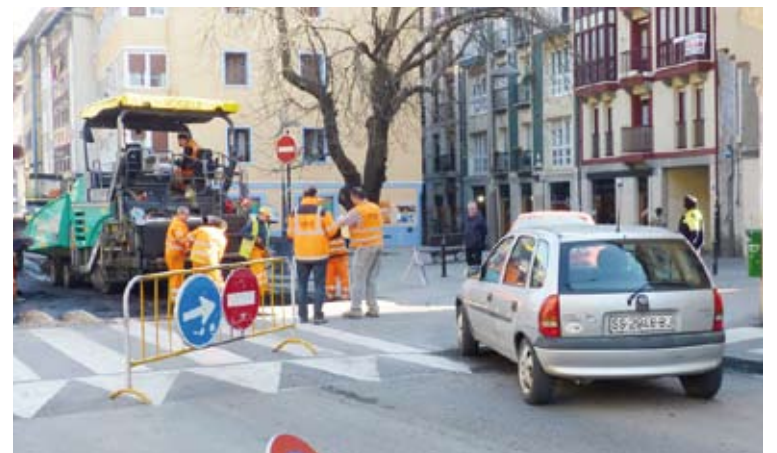
Asfalto-lanak Otalora kalean, Monterron parean. | U.M.
